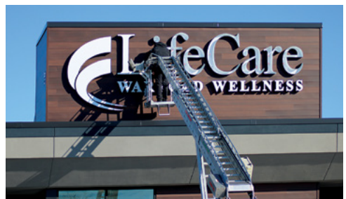
A sign crew installs LED lighted lettering along the rooftop of the all-new LifeCare Warroad Wellness facility in February.
